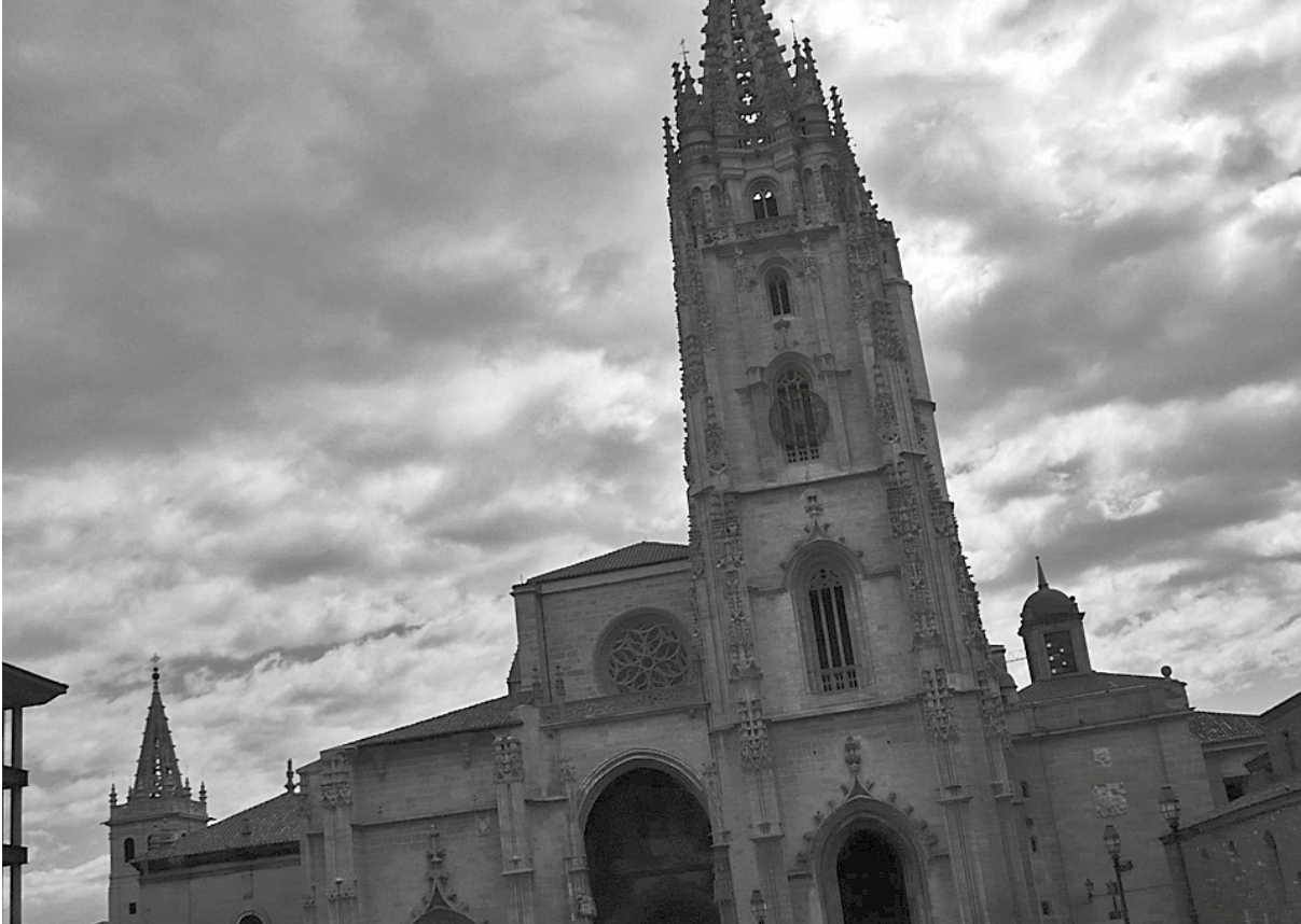
Fig. 1: Cathedral of Oviedo (Northern Spain) cleaned during 2000. The limestone façade shows no evidence of blackening in 2011.
