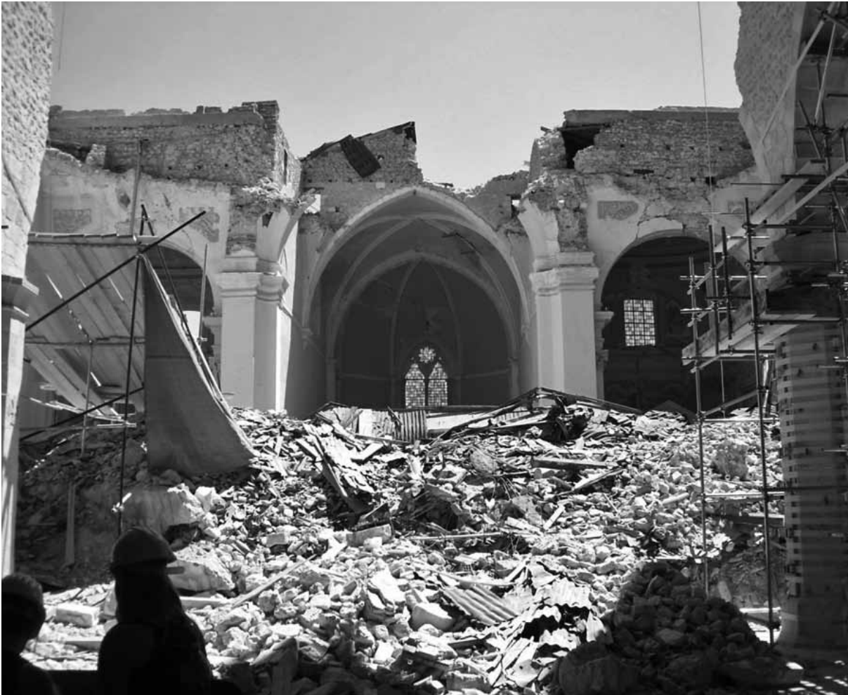
Fig.1: Damages produced in the earthquake 2009 in Abbey of Santa Maria Collemaggio in L'Aquila.
