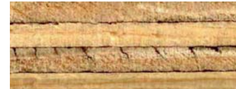
Figure 1.64: A magnified view of edge of a plywood showing tension checks (small splits).
