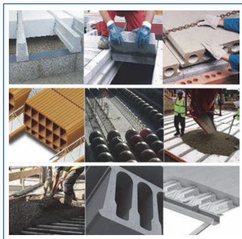
Figure 1.11. Examples of various precast, beam and block and in-situ composite separating floor types found in European countries. (left to right: full depth beam and block, shallow beam and block, hollowcore precast, in-situ beams with clay block infill, omni-floor system, lightweight insulated blocks with in-situ pour, deep profiled steel deck with in-situ concrete, deep hollowcore precast and shallow metal deck with in-situ concrete).
