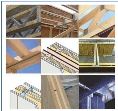
Figure 1.12. Examples of timber and lightweight frame wall and floor structures found in European countries. (left to right: open metal web joists, engineered I-joists, open timber web joists, solid joists, twin sheathed party walls, non-sheathed party walls, metal I stud twin party walls, cross laminated timber panels for walls and floors and metal C stud sections).
